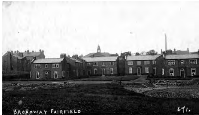
Broadway, during construction of houses c.1913-1920
