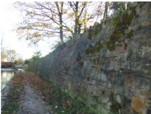
Stone wall adjacent to the canal towpath
