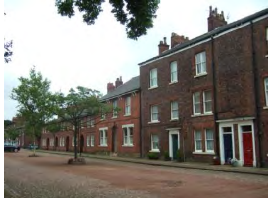
Numbers 21-38 Fairfield Square illustrates building facades of the 19 th Century
