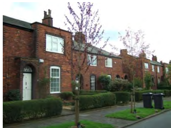
Houses on Broadway North
