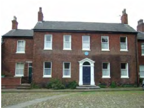
Former Doctors residence at 6 Fairfield Square
