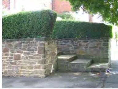
Stone retaining wall, hedge and steps at Broadway
