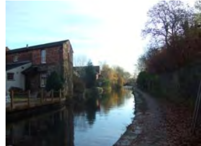
View adjacent to the canal bridge on Fairfield Road
