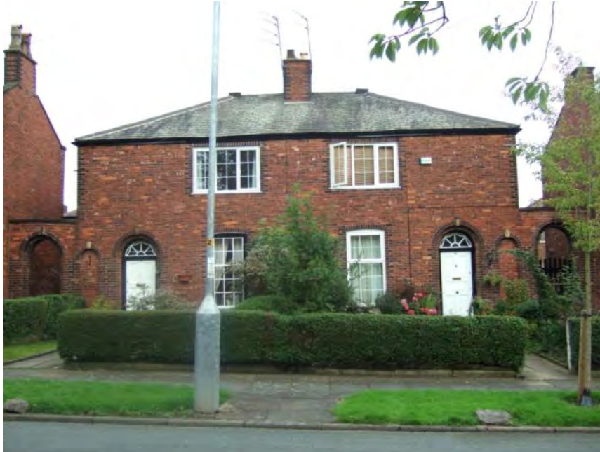
Houses on Broadway North with both original timber windows and doors and UPVC replacement windows
