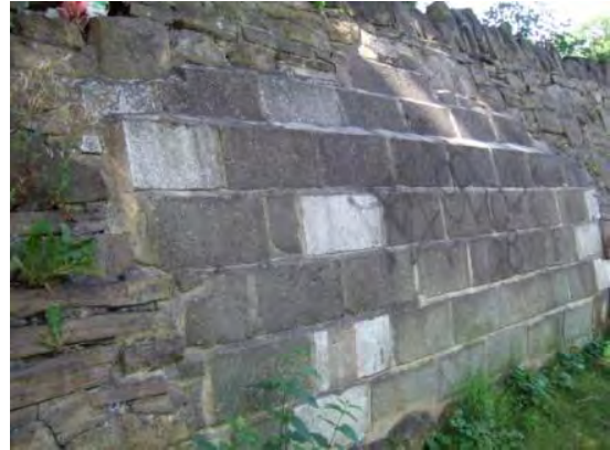
Area of block-work within the stone wall adjacent to the Canal.
