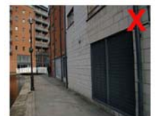
Blank facade at ground floor
