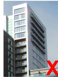
Protruding balconies appear to be an after thought
