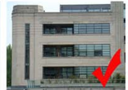
Recessed balconies complement the building's architectural style
