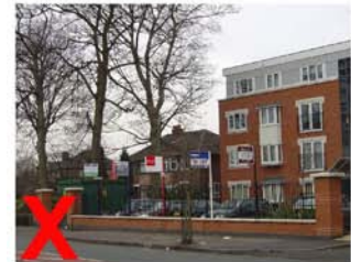
The scale, mass and architectural style of the flat block does not align with its two storey suburban surroundings
