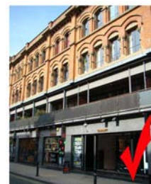
Simple detailing of the modern does not over dominate the historic
