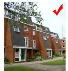
Primary entrances onto communal area
