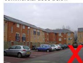
Large area of surface parking
