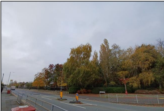
View of site taken from roundabout linking Greenside Lane, Chappell Road and Scott Road.
