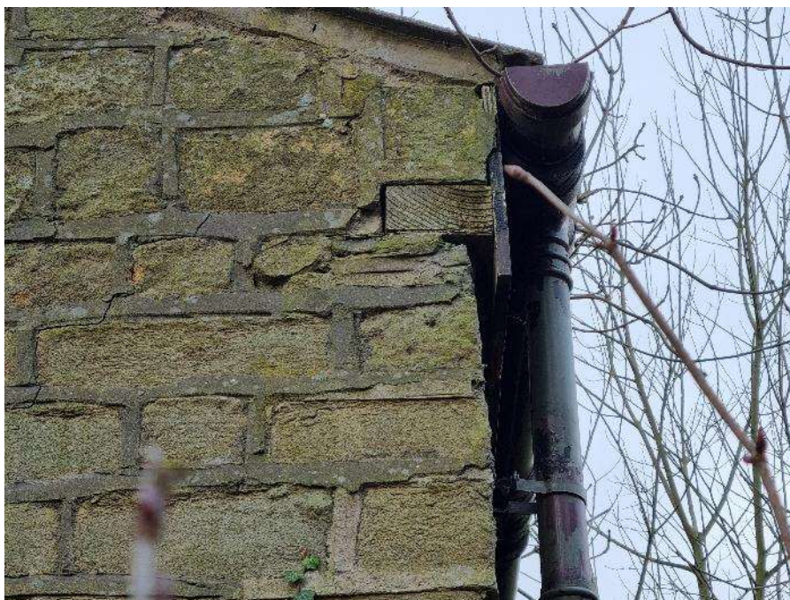
122. Exposed wall plate
