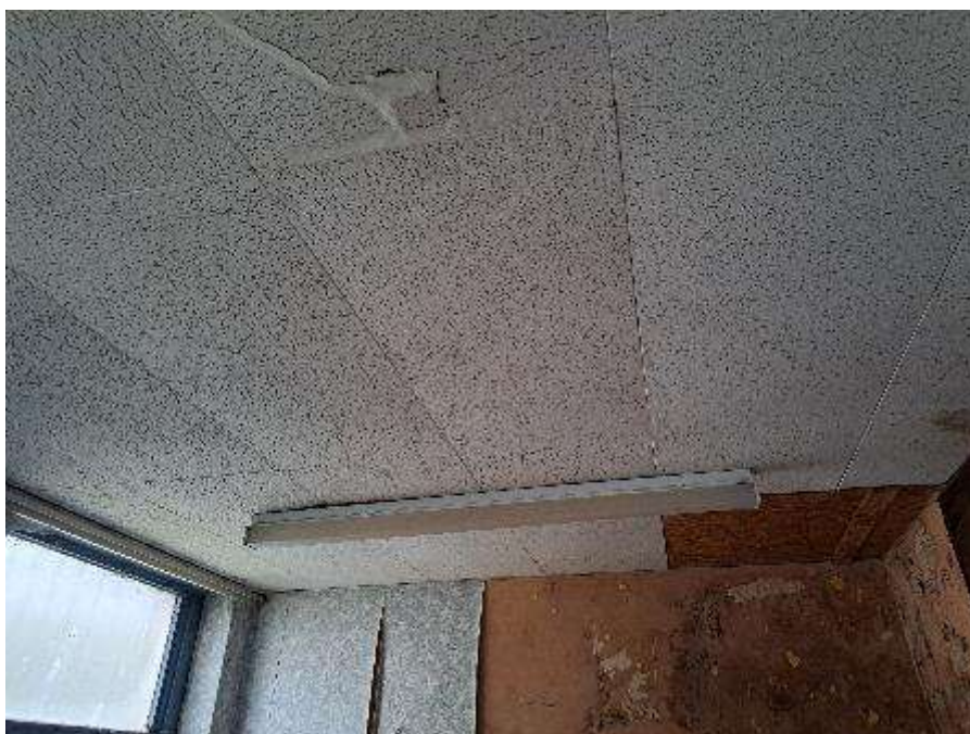
38. View of ceiling
