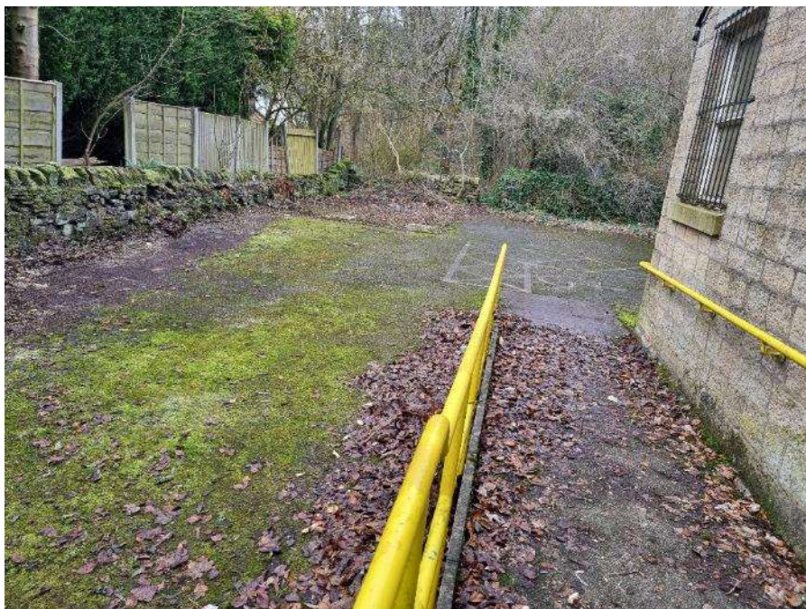
113. View of the ramp and surrounding areas.
