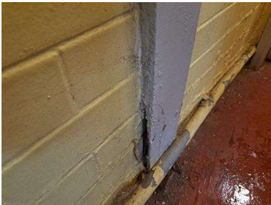
9. Damaged architrave
