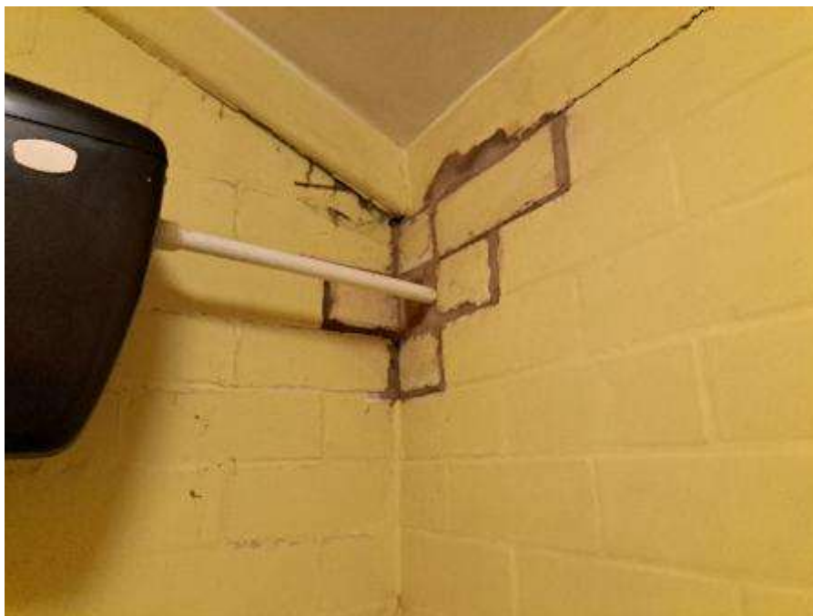
21. Cracking repairs
