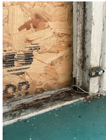
10) Rotten window frames – window fallen out
