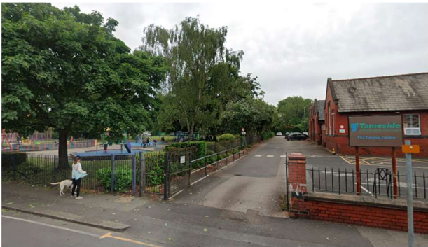
Existing Vehicular access off Acre Street
