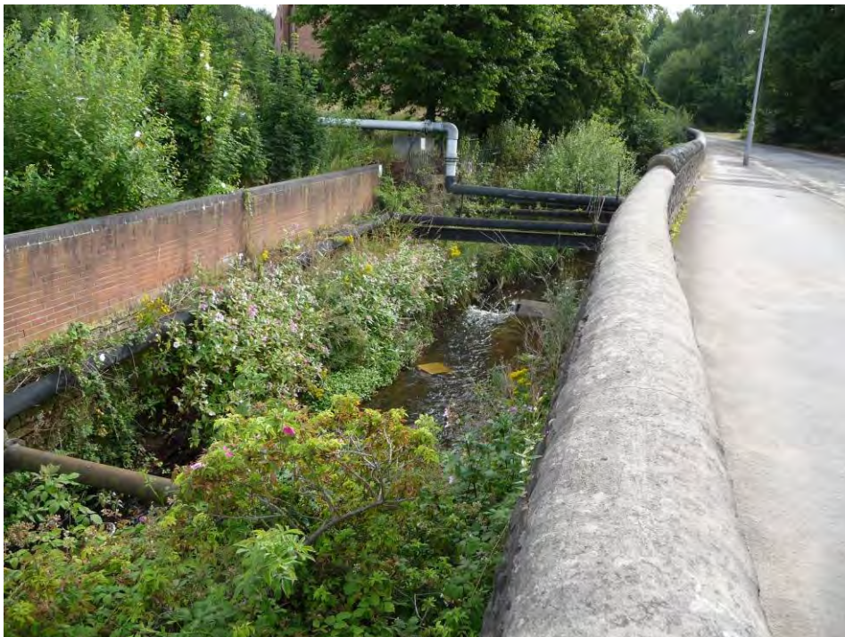
Plate 16 – View upstream adjacent to industrial estate
