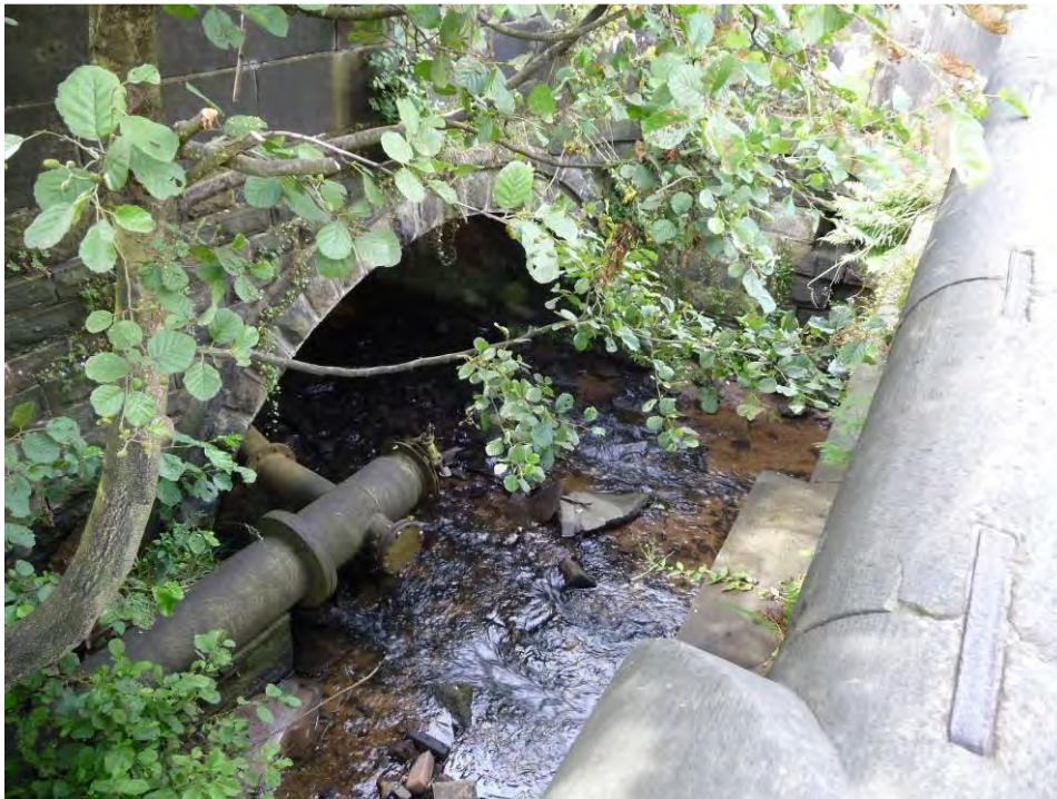
Plate 11 – Culvert inlet under Commercial Street
