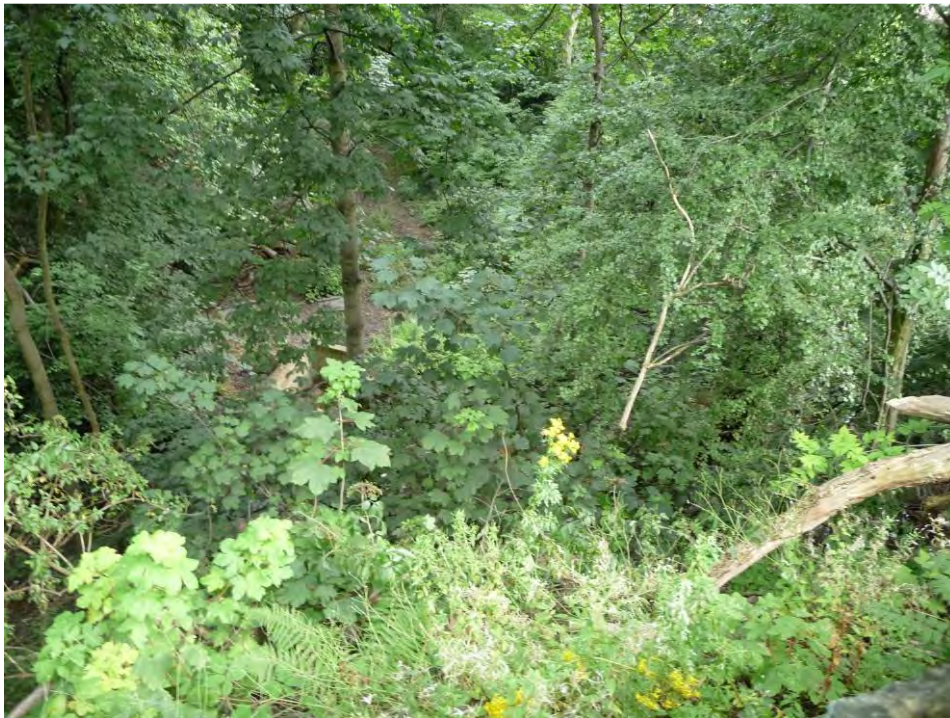
Plate 21 – View from Dukinfield Road of Wilson Brook on exit from culvert under Newton Street
