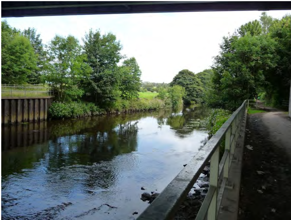
Plate 39 – View upstream from underneath M67
