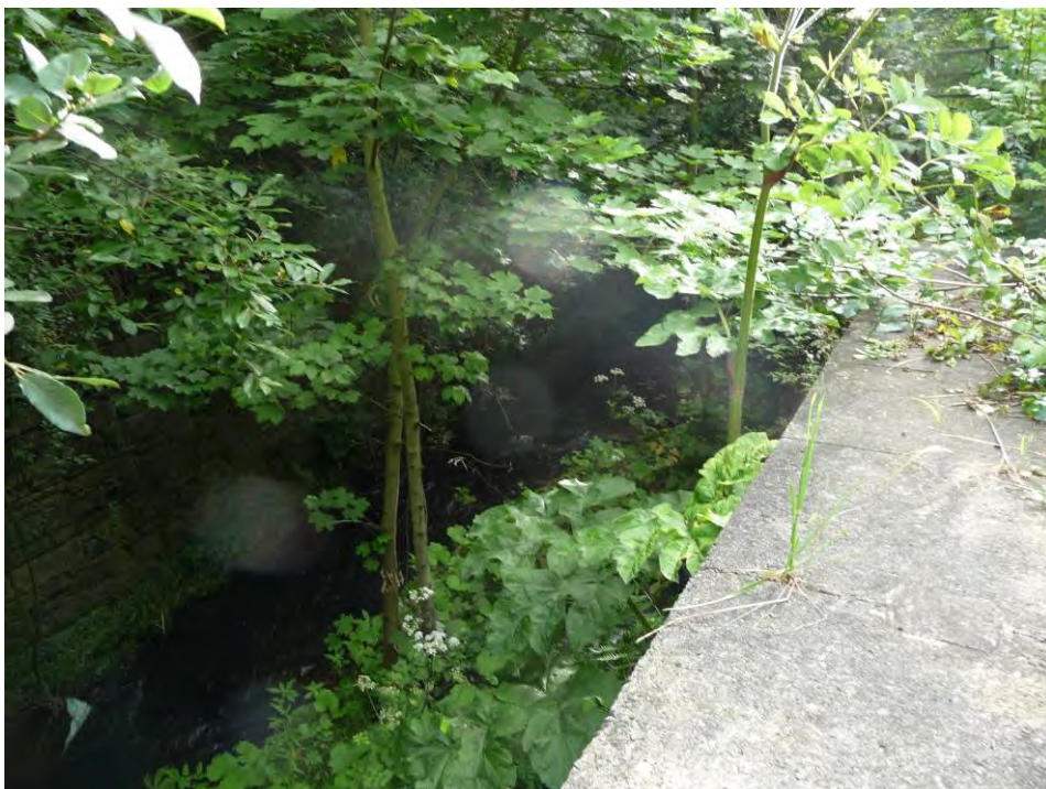
Plate 14 – View upstream of Godley Brook towards M67 culvert outlet
