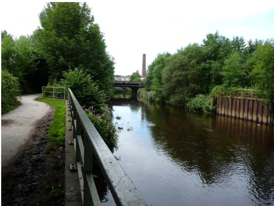
Plate 38 – View downstream from underneath M67 towards Manchester Road
