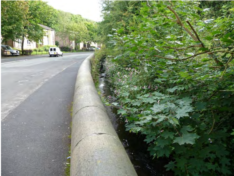
Plate 9 – View upstream along Wilson Brook from Commercial Street
