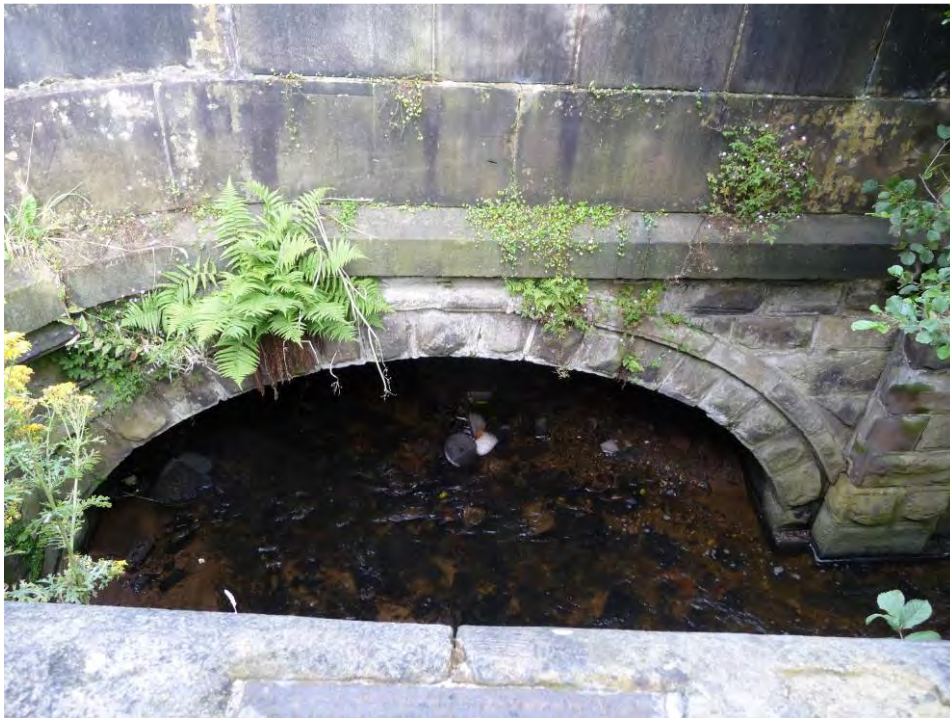
Plate 13 - Culvert inlet under Commercial Street
