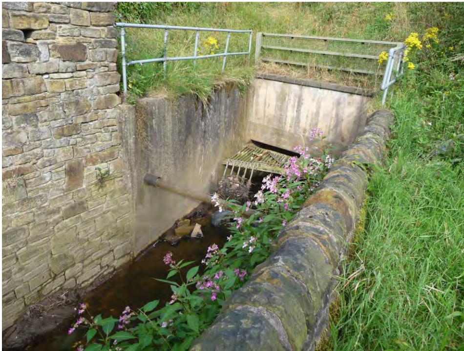
Plate 7 – Culvert inlet taking Godley Brook under M67
