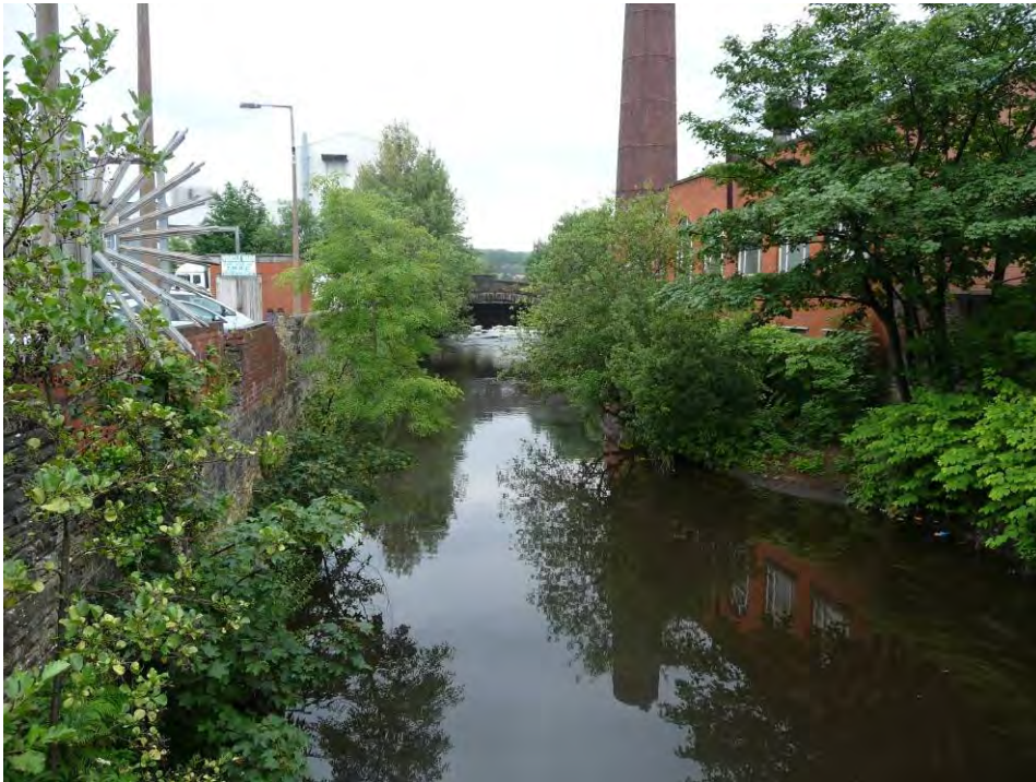
Plate 15 - View upstream from Tame Street bridge
