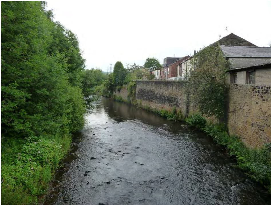
Plate 1 - View upstream from industrial estate vehicular access bridge off Northend Road
