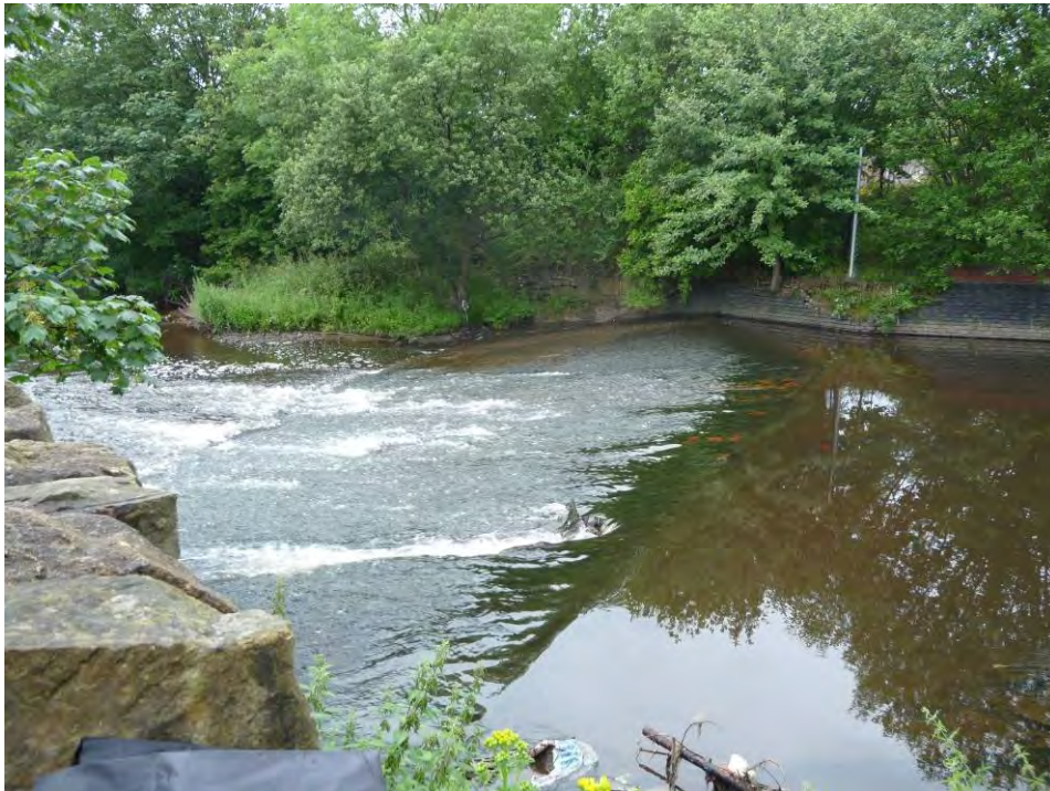
Plate 17 – Weir immediately downstream of Tame Street bridge
