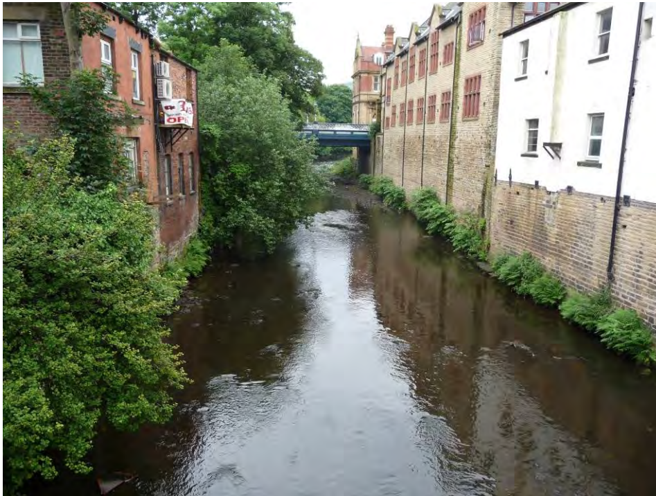
Plate 9 – View upstream from Melbourne Street bridge
