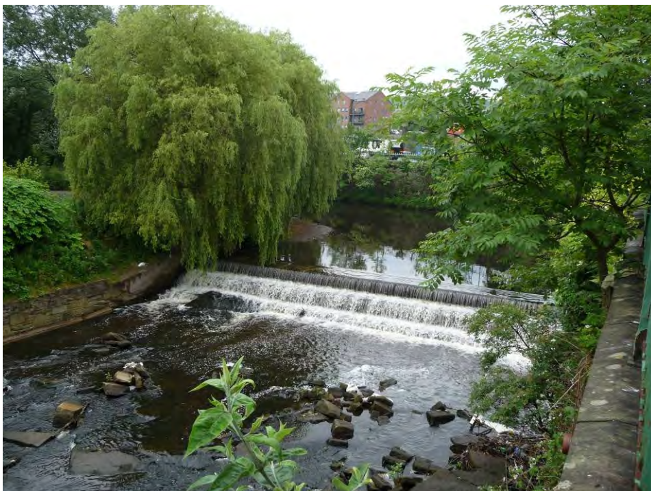
Plate 6 – Weir looking upstream from Corporation Street
